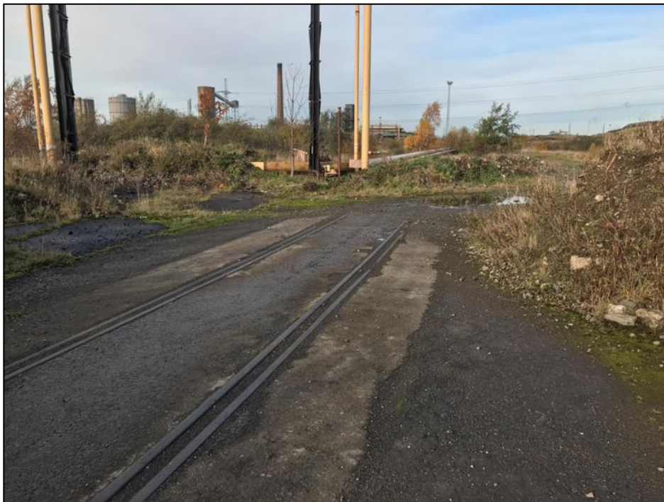
Figure 7-1 – Example of mixed permeable and impermeable surface with evidence of significant previous use/development
